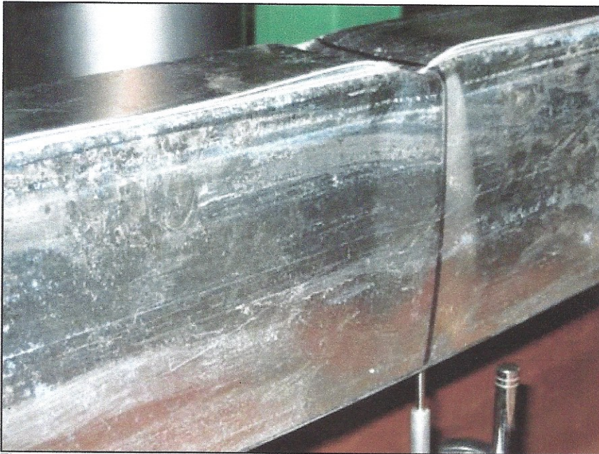
Figure 4 - Flange at Failure at Mid-Span
